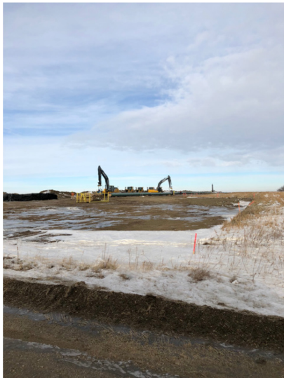
17. Prep Crew – 168km+900 – Dec 1, 2017
