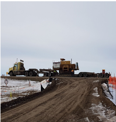
5. Hydro vac – Km 159+450 – Nov 28, 2017
