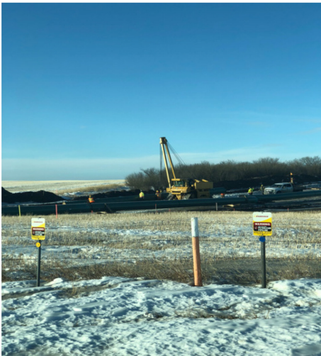
3. Set up crew (East) – km 161+650 – Nov 25, 2017
