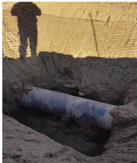
12. Prep Crew - 159km+400 – Nov 30, 2017
