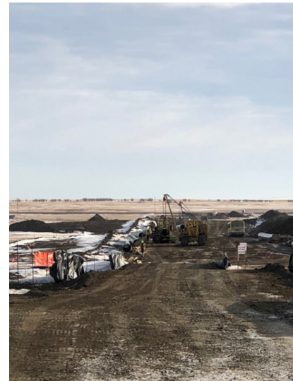
18. Bending Crew – 169km+700 – Dec 1, 2017
