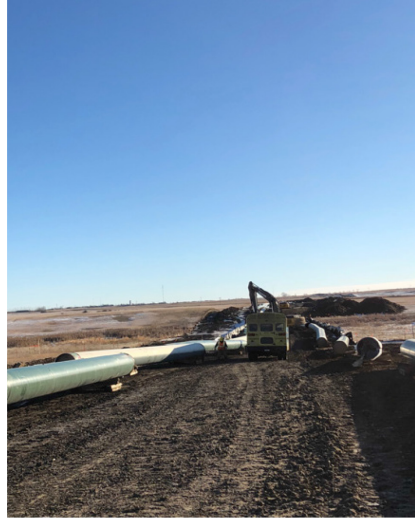
14. Prep crew (S.E) – 165km+550 – Nov 30, 2017
