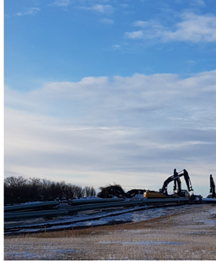
2. Set up Crew – Km 161+600 – Nov 27, 2017
