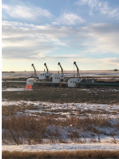
20. Mainline Crew – 166km+600 – Dec 2, 2017
