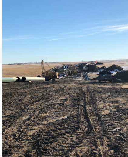
8. Bending Crew – Km164+500 – Nov 28, 2017
