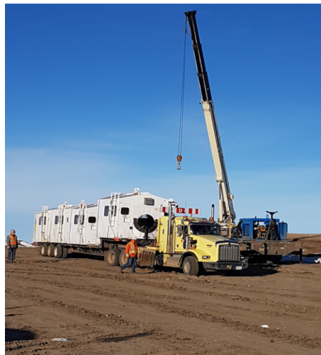
6. Welding Crew – Km 159+350 – Nov 28, 2017
