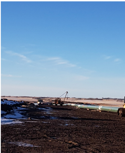
9. Bending Crew - km167+500 – Nov 29, 2017
