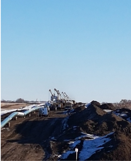
13. East of clean-up - 161km+900 – Nov 30, 2017
