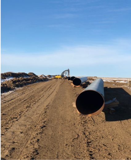
7. Prep Crew – Km 162+900 – Nov 28, 2017
