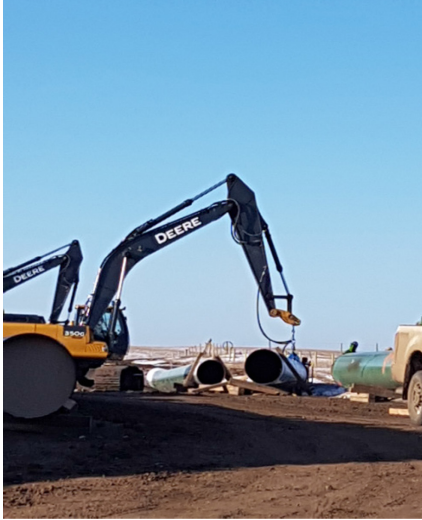
1. Prep crew – km 160+400 – Nov 27, 2017
