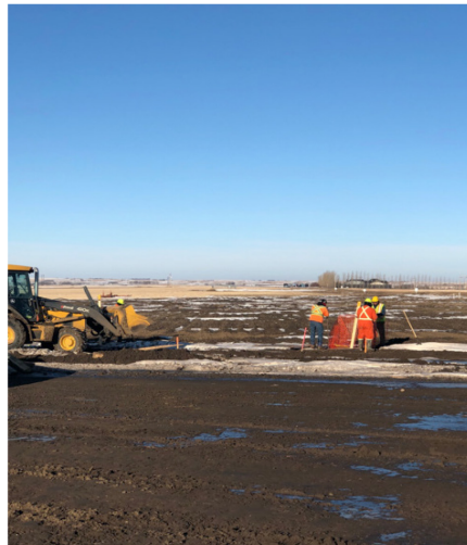
4. Hydrovac site hole backfill – Km 167+500 – Nov 27, 2017
