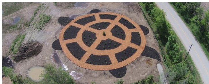
> Healing garden at Dawn Storage facility in Ontario.
