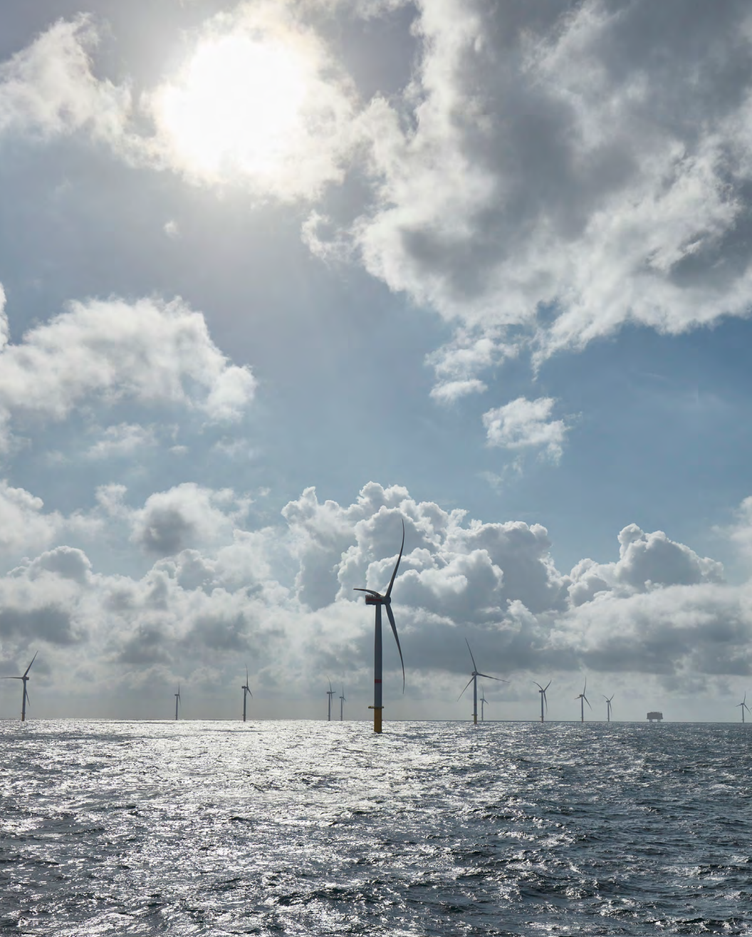
> The 497-MW Hohe See offshore wind project, in the North Sea off the coast of Emden, Germany.
