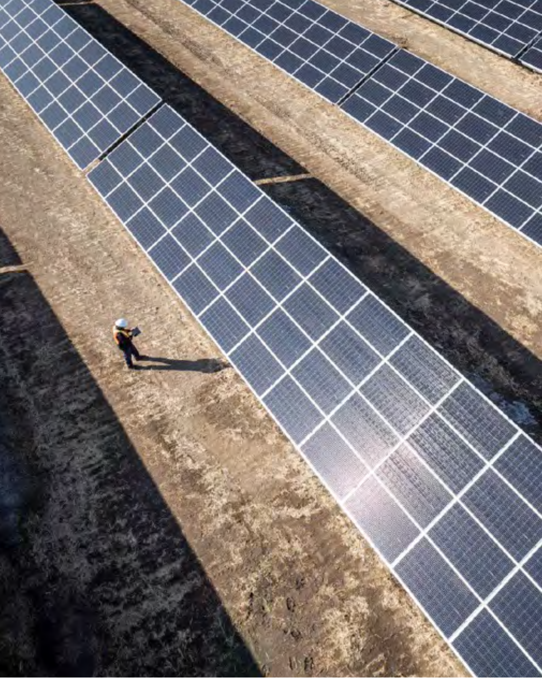
> Alberta Solar One is part of Enbridge's growing solar portfolio.
