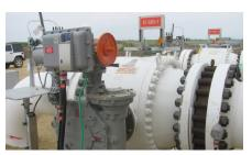
Motor operated ball valves allow our control staff to remotely close sections of our pipelines immediately upon detection of a potential issue.
